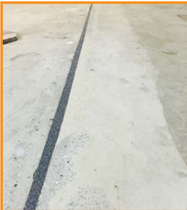
Installation of PNSX™ at Westfield Carindale to repair spooled concrete and expansion joint rebate. The CPSX™ carpark expansion joint system has also been installed (see the CPSX™ data sheet for further information about this product).
