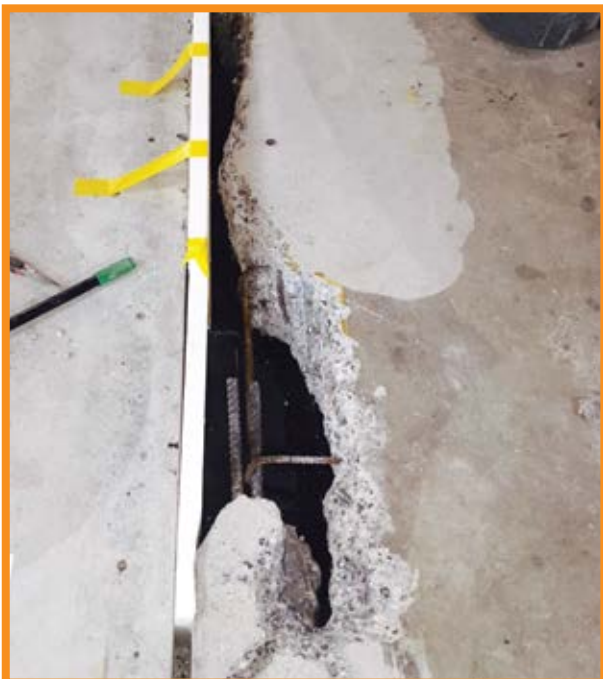
Installation of PNSX™ at Westfield Carindale to repair spooled concrete and expansion joint rebate. The CPSX™ carpark expansion joint system has also been installed (see the CPSX™ data sheet for further information about this product).
