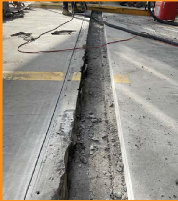
Installation of PNSX™ to car park ramp at Pacific Fair Shopping Centre to repair spooled and broken concrete. CPSX™ was also installed.
